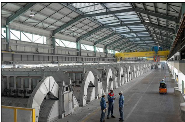
Figure 1. Longest electrolysis potline with DX+ cells operating at 470 kA. EGA, Abu Dhabi
